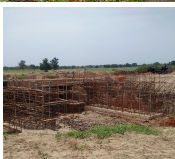
3-CELLS CULVERT ON MAIGANGA ROAD, GOMBE STATE
